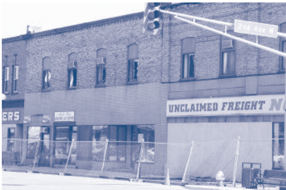
The most recent site of a fire
